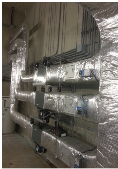
Hydroxyl generators were used in the HVAC system for chemical dosing rooms.
